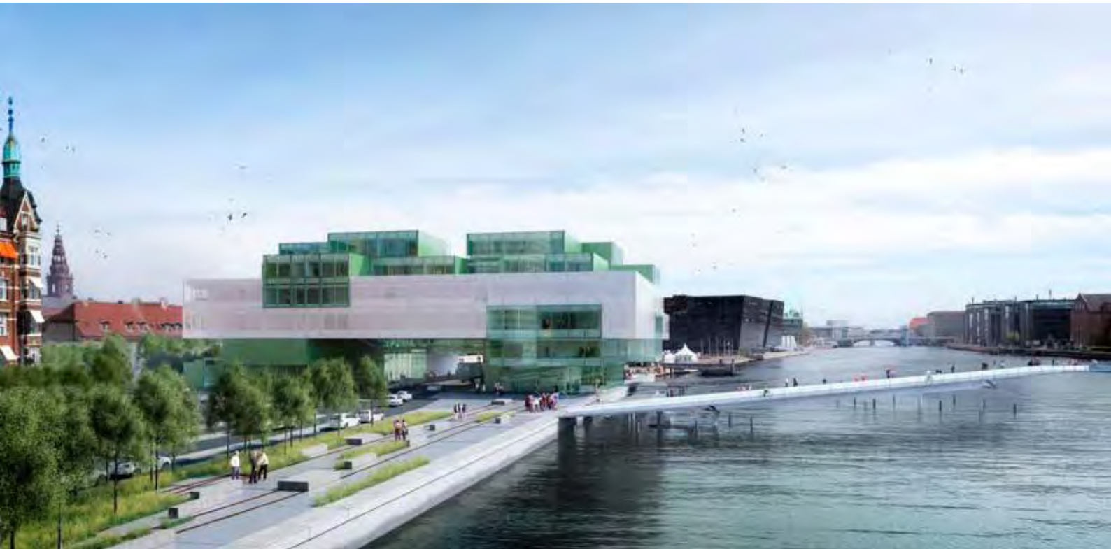
Western bridge abutment
