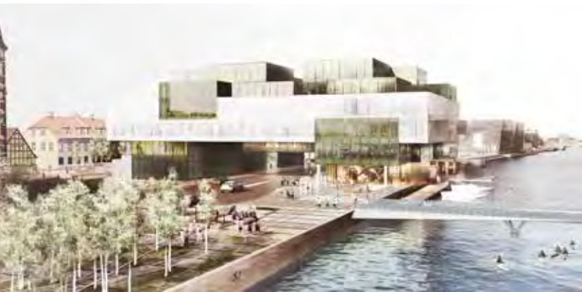
Western bridge abutment
